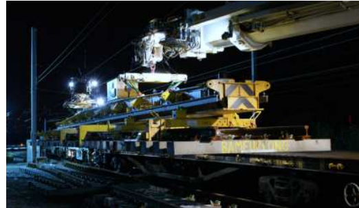
Figure 12: Kirow with adjustment beam between jib and lifting beam. [Network Rail]
